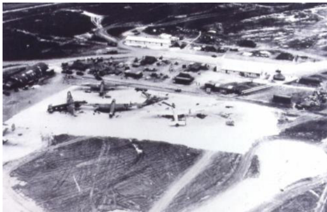
Maintenance Area at Torretta Field, Italy
